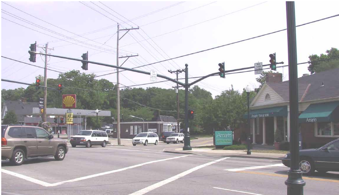
Example of mast arm traffic signals: Madeira, Ohio
